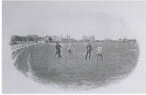
The Road Hole in the 1890's. The only building still standing is the Station Master's house now the Jigger Inn.
