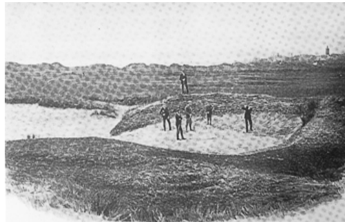
Hell Bunker - one hundred years ago
